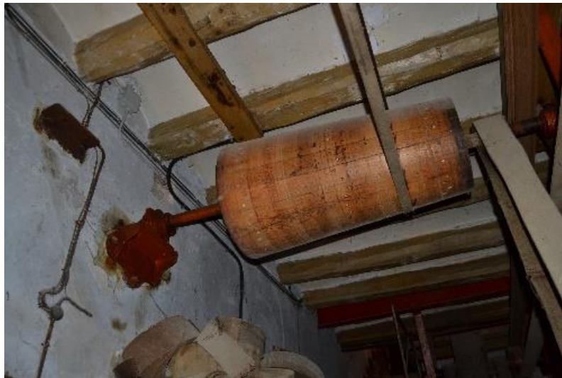
Wheels and transmission mechanisms on the ground floor of the mill149
