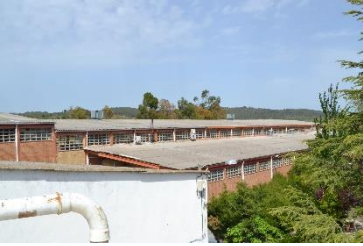
View of the factory in the northeast direction.
