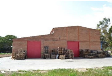
East view of the work warehouse.
