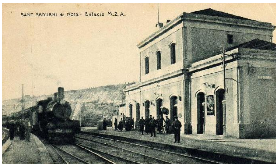
View of the station of Sant Sadurní D'Anoia at the end of the nineteenth century. 131
